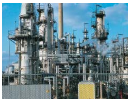
Cleaning Boiler, Condenser, Heat Exchanger & Piping in Chemical Process Industries
